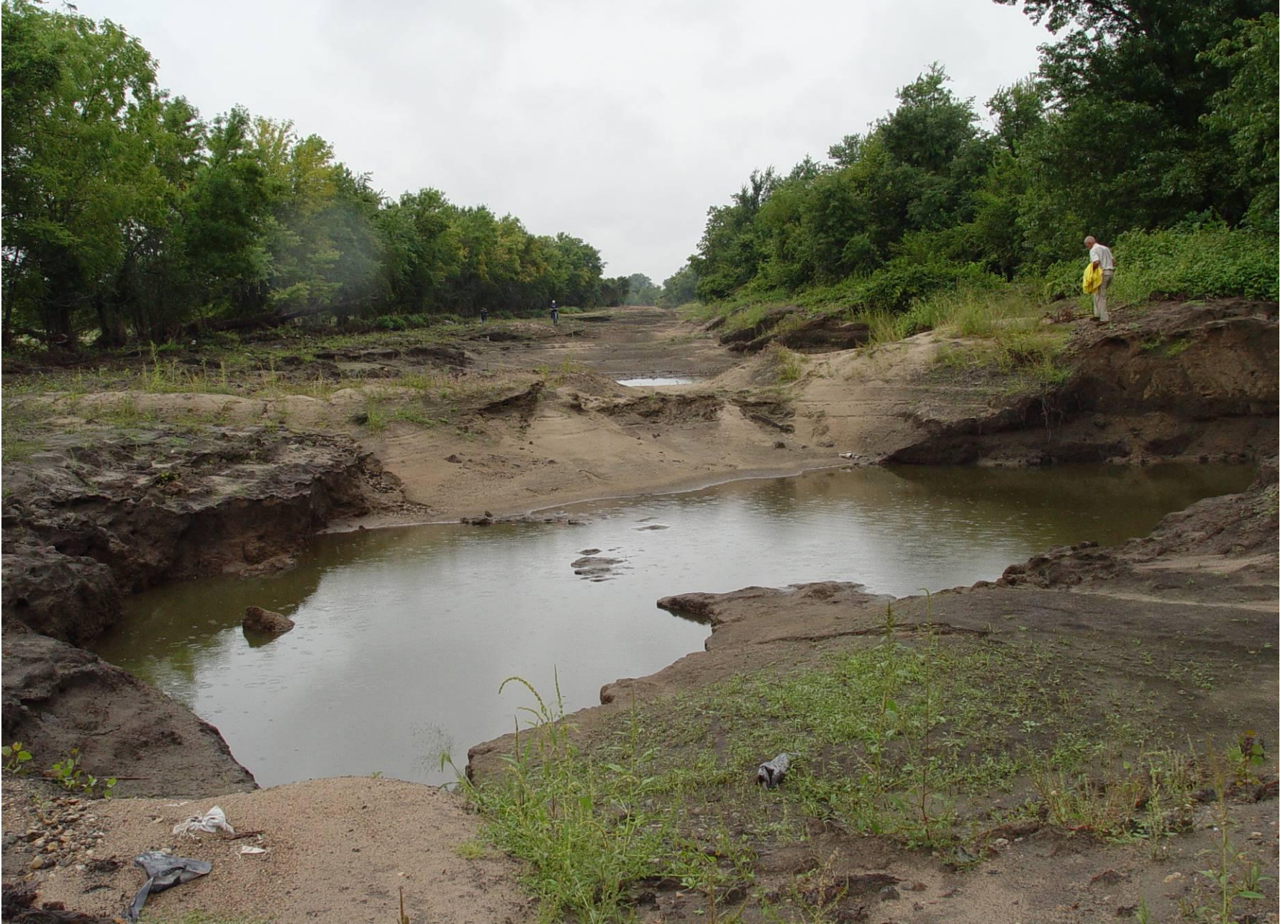
Scour holes in a shale foundation testified to a large volume of water sweeping through, leaving almost no trace of the levee behind
